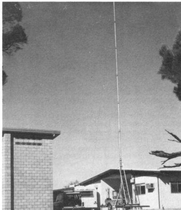
The 60ft. pump-up St. John temporary radio mast.
